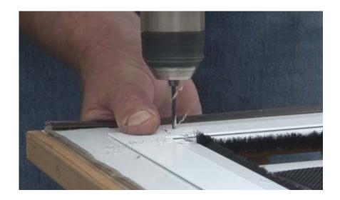
10. Using the included bit, approximately 1" in from the overlapping flange ends, drill and secure the pet door frame to your screen door and fasten with provided screws. Do not drill completely through your screen door frame.
