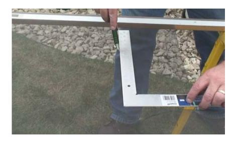
6. Cut screen from Point A to Point C using a straight edge and utility knife.
