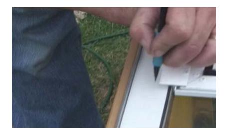
3. Mark the horizontal screen cut location on the sliding screen door frame with a pencil. It is best to mark the cut location a 1/8" in from the end of the H channel (Overlay flange) attached to the Pet screen door to allow enough screen material to roll into Pet Screen Door Spline groove. (Point A)
