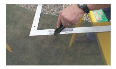
7. Cut screen from Point C to Point B using a straight edge utility knife.
