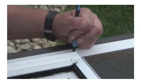
4. Make the same mark at the bottom corner of the overlay flange - bottom corner of your screen pet door; 1/8" in from the end of the H channel. (Point B)
