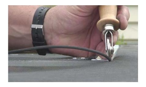
12. Repeat same process from Point C to Point B. Keep the screen taunt by applying constant pulling pressure to ensure a tight fit.
