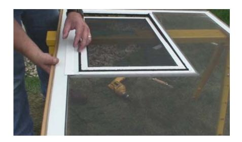
9. Position the Security Boss® screen pet door over the cut opening. Pet door should be firmly seated into the corner of your sliding screen door.
