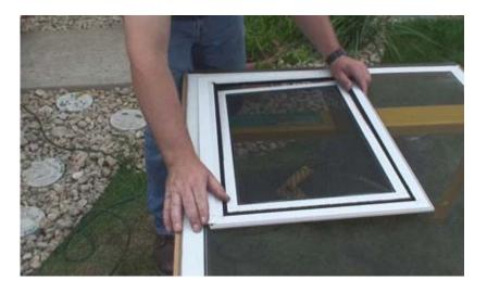
2. Position the pet door on your screen door, spline grooves up. The pet door must be mounted in the bottom corner. For example, most patio screen doors have the screen spline groove to the exterior; the Pet screen door spline groove should therefore be to the exterior as well.
