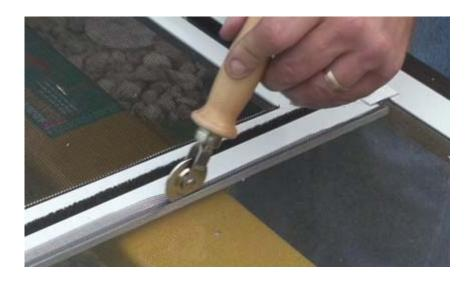
11. Using the included roller tool and spline, start at Point A and attach the screen to the pet door frame moving towards Point C
