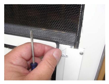
Clip two metal retainers over the pet screen door raceway. One retainer must be positioned as close the unsupported pet screen door corner as possible. The other can be spaced along the raceway
