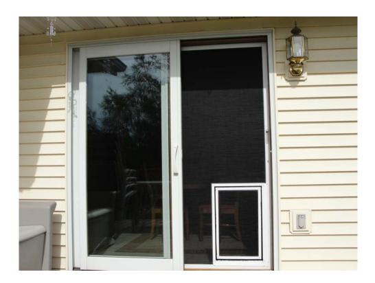
Measure the distance between the vertical frames of the patio screen door the pet door is installed into. Measure from the side that does not have the screen spline cord visible. This distance will be the length you will cut the Brace Bar to. Mark this distance on the Brace Bar.
