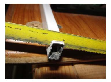
Test the fit of the brace bar between the patio screen frame rails. Re-cut if needed.
