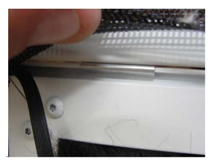
Once the metal retainers are positioned on the raceway, side the brace bar down to within 1/16" of touching the pet screen door. The brace bar should be resting along the top edge of the pet door screen frame and between the screen fabric and tab of the metal retainer that has a hole.
