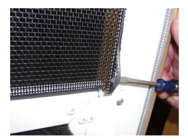
Insert the brace bar retainer clips into the brace bar. Leave enough of the retainer clip out of the brace bar so it can clip onto the patio door screen frame raceway.
