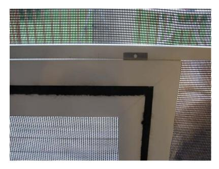
Push the screen spline back into the raceway on the Pet screen door; be sure to keep the screen fabric snug as you are rolling the spline in to the raceway.
