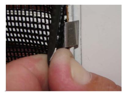
Push the screen spline back into the patio door raceway to secure the brace bar clips. Be sure to keep the Screen fabric snug as you are rolling the spline into the raceway
