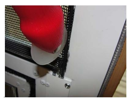
Remove the screen spline that is securing the top of the Pet screen door (if previously installed).
