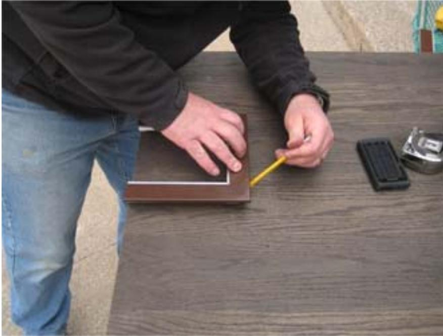
**Step 5—WOOD DOORS:** For wood doors, drill out two corners diagonal from each other using a 7/8” paddle bit or a 5/16” regular bit. If you use a regular bit, drill three holes close together then elongate the holes until you have connected the three holes. This will allow insertion of the reciprocating saw blade. Cut out the rough opening along the traced lines.
