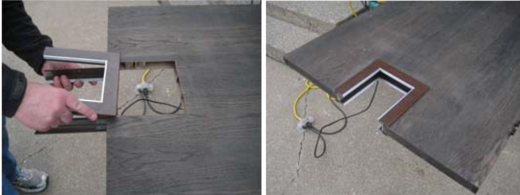
**Step 8:** Using the pre-drilled pilot holes and supplied drill bit, drill and insert one screw into one leg of the Pet Pass Thru Cat door so that it anchors in the solid wood along the bottom edge of the door (As Mentioned in Step 3) Make sure the door is level. When level, tighten the inserted screw. Repeat with other leg of cat door. Affix remaining screw into place using the pilot hole as guide.
