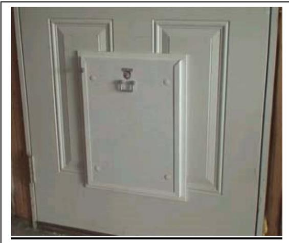
**Step 10:** The Insulated Security panel will slide into place and fasten with the dead bolt lock.
