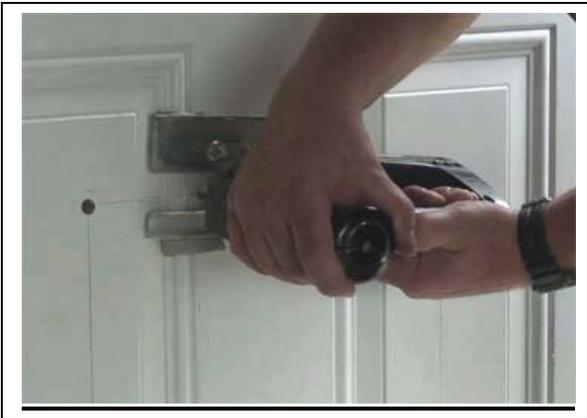
**Step 5:** METAL DOORS: For metal doors, follow the above directions for wood doors, using an appropriate blade made for cutting metal.
