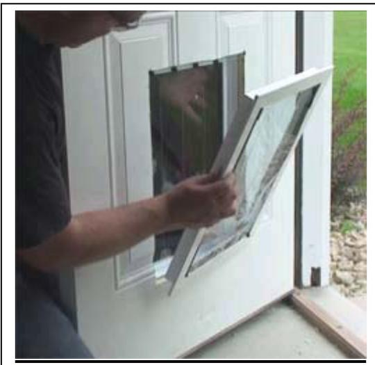
**Step 6:** Separate the Interior and exterior door frames. Remove the Insulated Security Panel from the inside frame.
