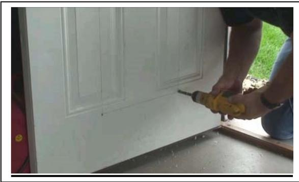
**Step 5:** WOOD DOORS: For wood doors, drill out two corners diagonal from each other using a 7/8" paddle bit or a 5/16" regular bit. If you use a regular bit, drill three holes close together then elongate the holes until you have connected the three holes. This will allow insertion of the reciprocating saw blade. Cut out the rough opening along the traced lines.
