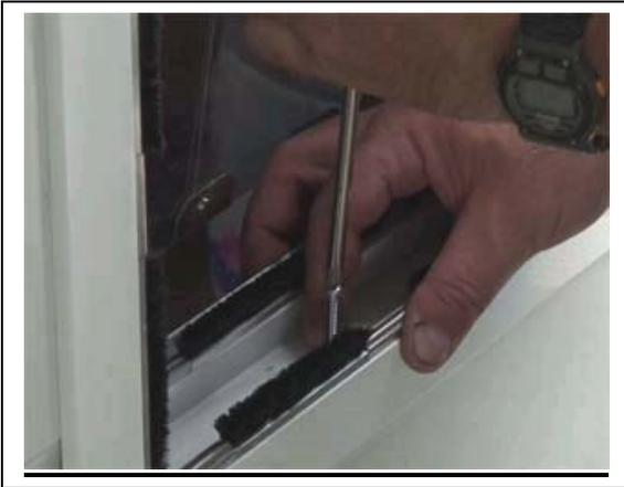
**Step 8:** Using the pre-drilled pilot holes and supplied drill bit, drill and insert one screw. Make sure the door is level. When level, tighten the inserted screw. Affix remaining screws into place using the pilot holes as guides.
