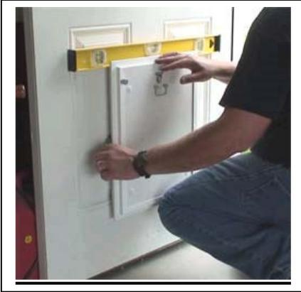
**Step 4:** Trace the flange of the MaxSeal® door using a pencil. Use the dimension of the flange perimeter to determine the dimension of the rough opening.
